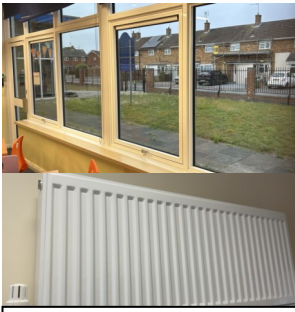
Some of the building work at St Teresa's
